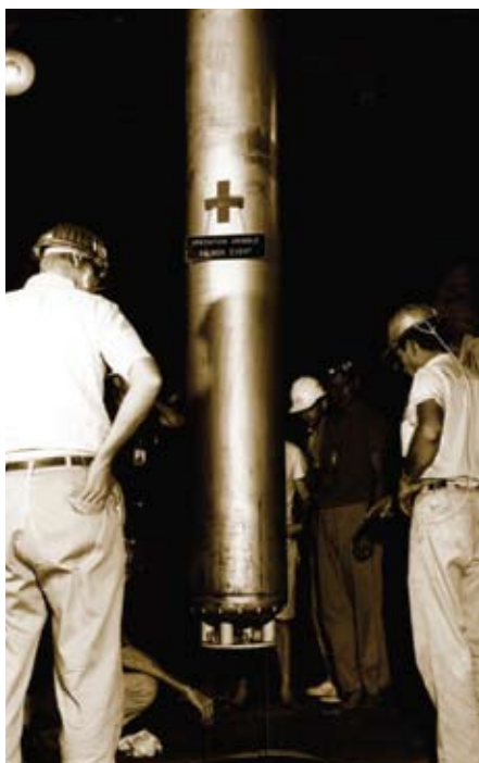
THE 1964 SALMON EVENT, A FIVE KT DETONATION CONDUCTED 280 METRES DEEP IN A MISSISSIPPI SALT DOME, CONFIRMED THE THEORY OF DECOUPLING AS A MEANS OF CONCEALING CLANDESTINE NUCLEAR EXPLOSIONS. IN THIS PHOTO, EXPERIMENTERS ARE LOWERING A CANISTER CONTAINING THE NUCLEAR EXPLOSIVE FOR THE SALMON EVENT.
