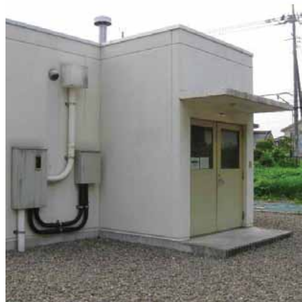
Radionuclide station RN38, Takasaki, Japan
