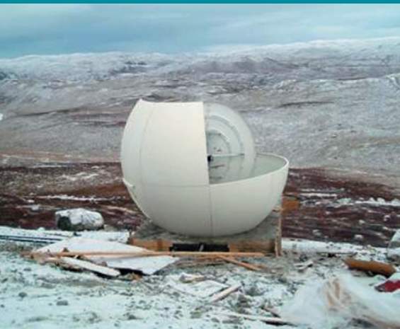
Station AS27, Sondre Stromfjord, Groenland (Danemark).
