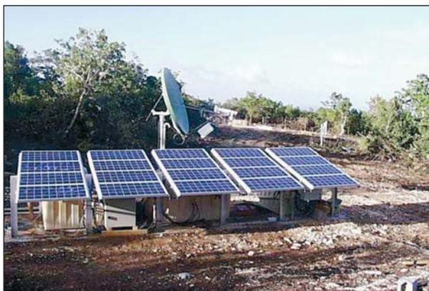
1. Solar panels, battery packs and satellite dish at the southern element of HA5, Guadeloupe (France), the first T phase hydroacoustic station to be certified (January 2002).
