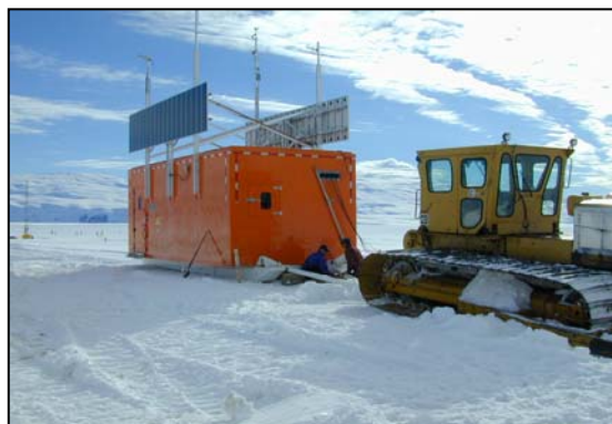
MOVING THE HYBRID DIESEL/SOLAR POWER SUPPLY UNIT AT WINDLESS BIGHT
