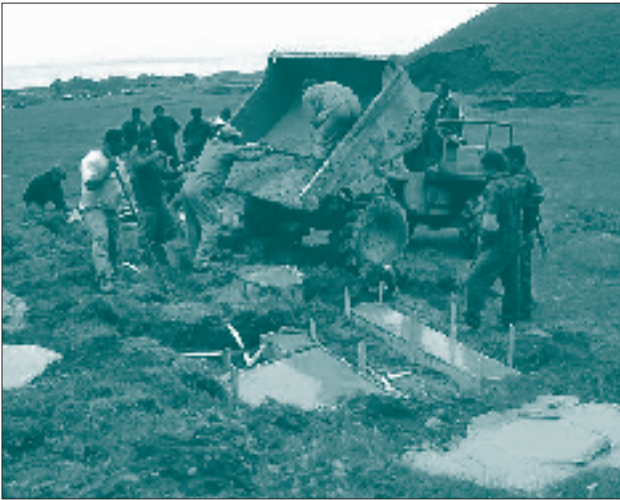
ISLANDERS HELPING TO BUILD INFRASOUND STATION IS49
