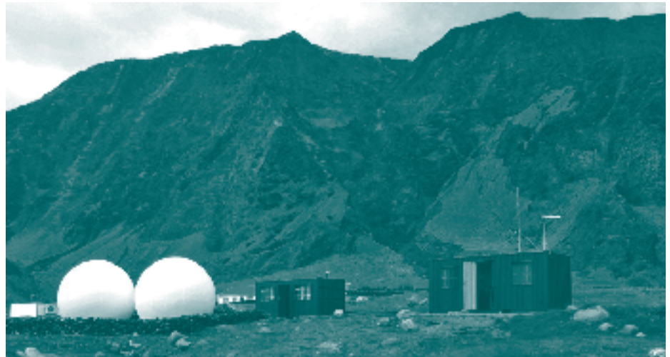
CENTRAL PROCESSING FACILITY (CPF) AND RADOMES, TRISTAN DA CUNHA
