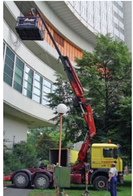
CRANE MOVING UNINTERRUPTIBLE POWER SUPPLY TO THE NEW PTS COMPUTER CENTRE
