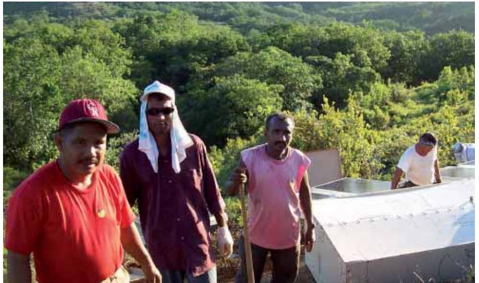
PALAUAN WORKERS CONSTRUCTING THE REPEATER SITE OF INFRASOUND STATION IS39, PALAU
