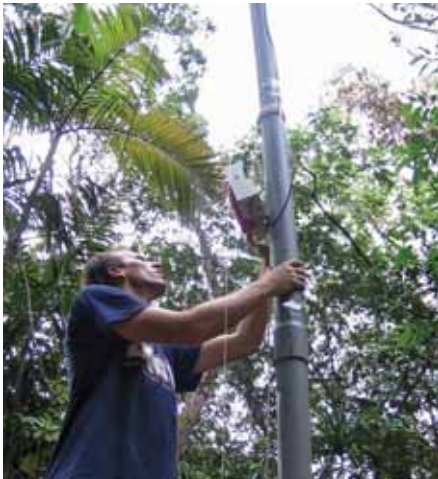
FIXATING 11 METRE HIGH PLASTIC TUBE WITH ANTENNA ON TOP FOR DIFFERENTIAL GPS MEASUREMENTS
