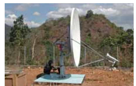
INSTALLATION OF GCI ANTENNA, AS44, KAPPANG, INDONESIA, NOVEMBER 2002
