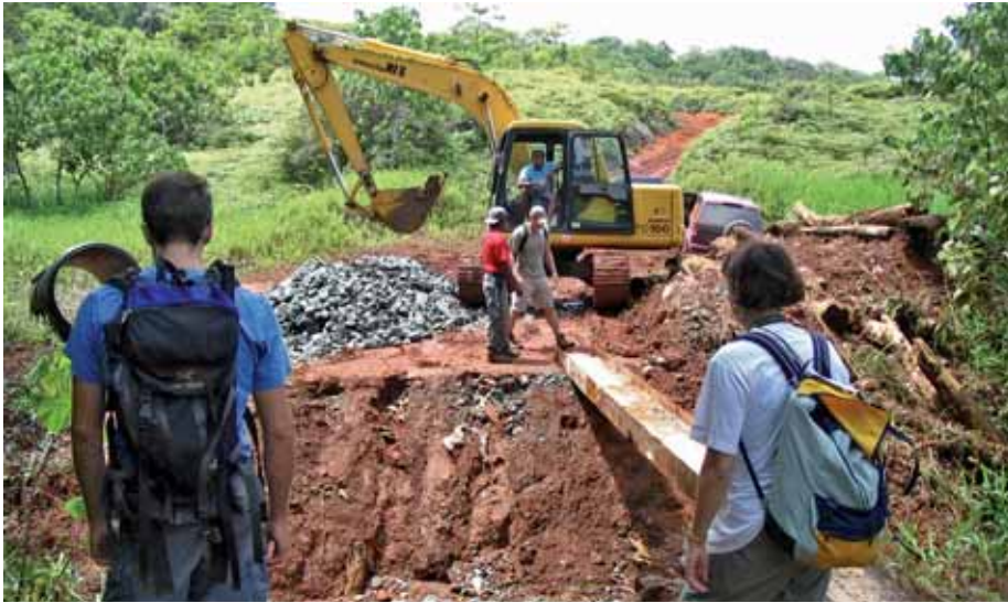
CERTIFICATION TEAM USING U-BEAM TO ACCESS INFRASOUND SITE WHILE BRIDGE IS BEING RECONSTRUCTED, PALAU, JUNE 2005
