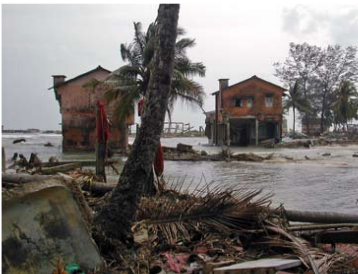
DEVASTATION CAUSED BY 2004 TSUNAMI, MALACCA VILLAGE, SRI LANKA
