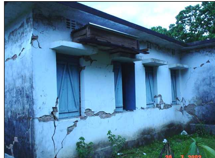
2003: Brick Masonry Building, Kolabunia
