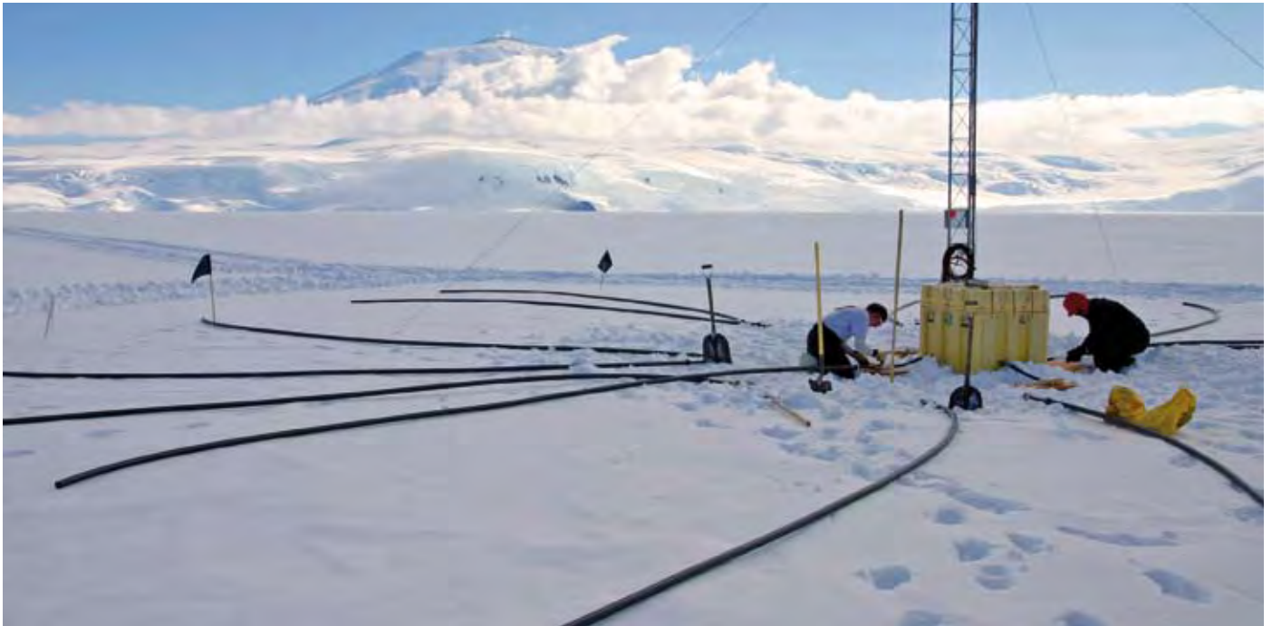
RE-ATTACHING WIND NOISE REDUCTION PIPE ARRAY TO VAULT AT IS55. PHOTO COURTESY OF DUNCAN MARRIOTT, GEOPHYSICAL INSTITUTE, UNIVERSITY OF ALASKA, FAIRBANKS.
