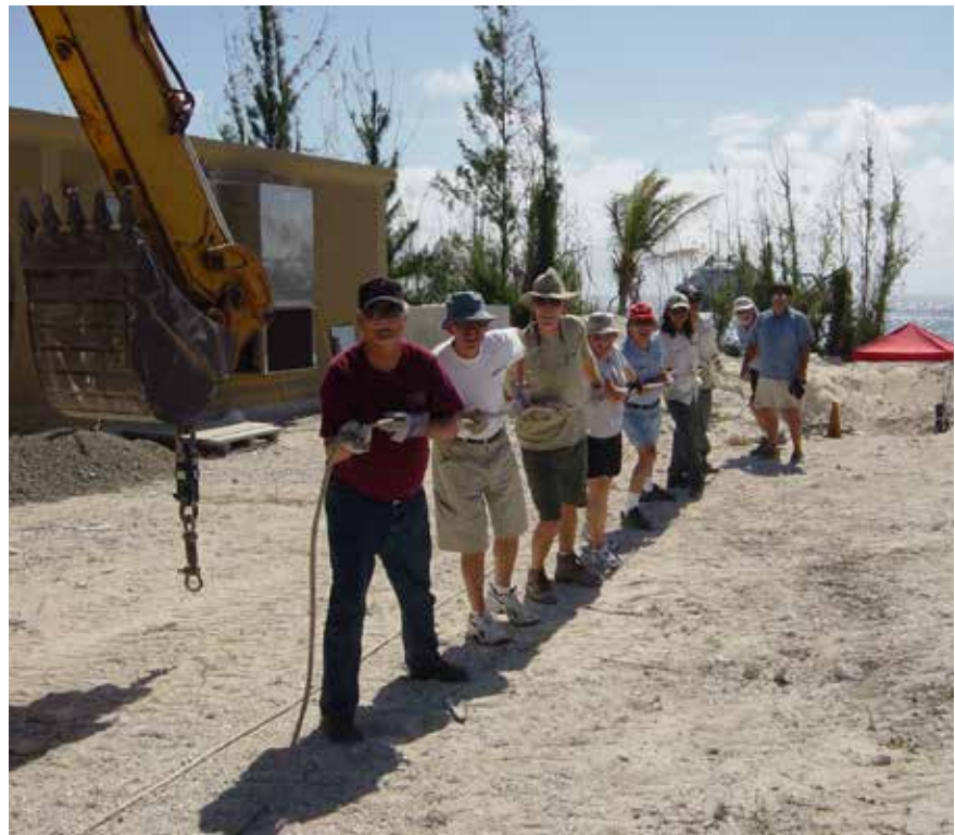
Installation of hydroacoustic station HA11, Wake Island, USA.
