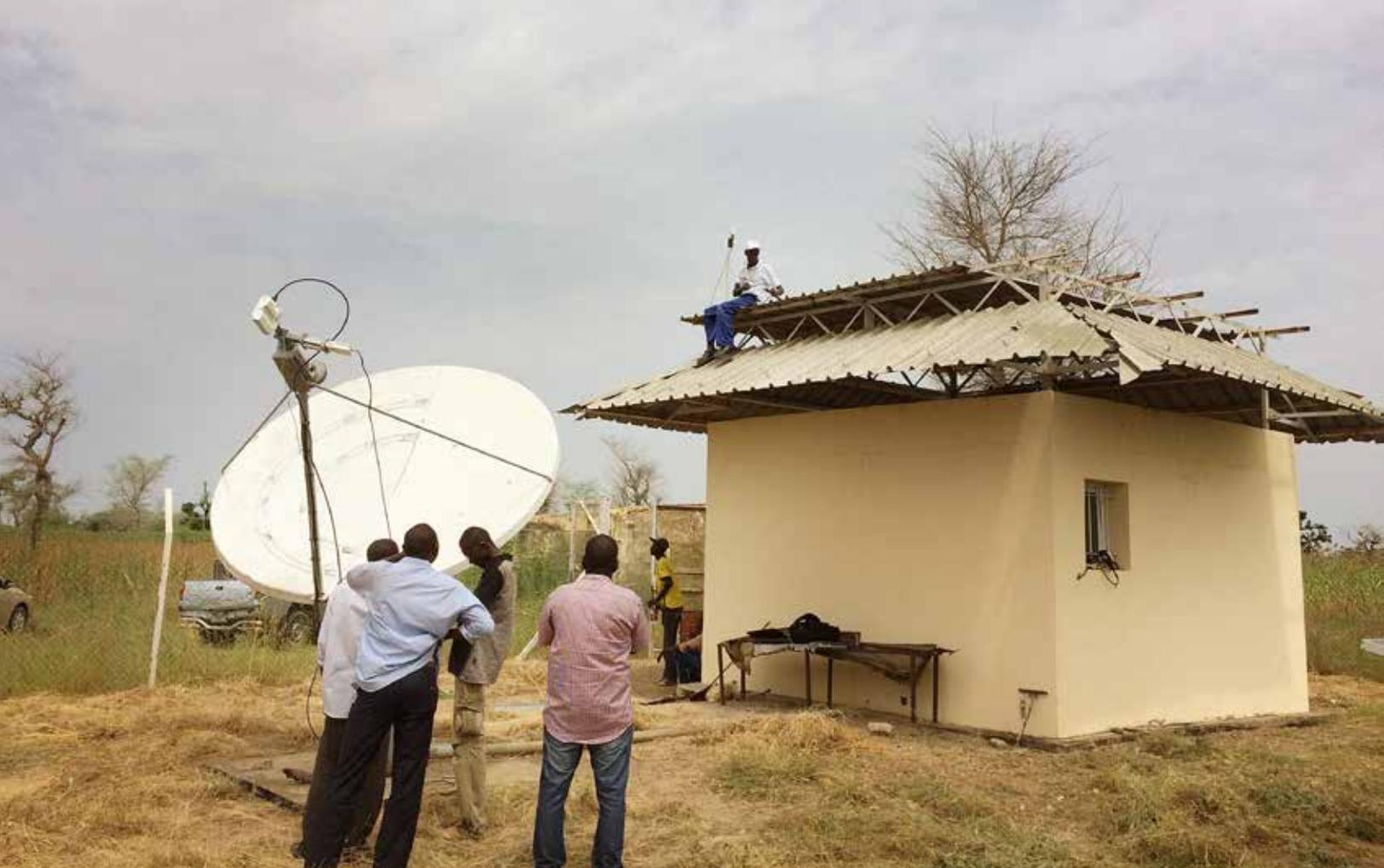
*A team of technicians working to fix the VSAT antenna. In the background an operator is installing the GPS receiver.*
