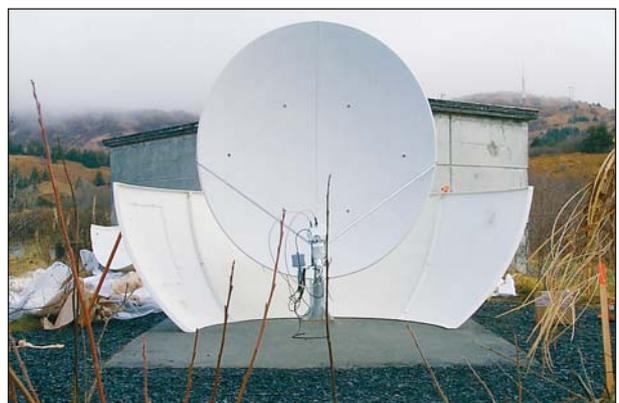
*Installation of a VSAT antenna in a radome at auxiliary seismic station AS110, Kodiak Island, Alaska, USA, December 2002.*
