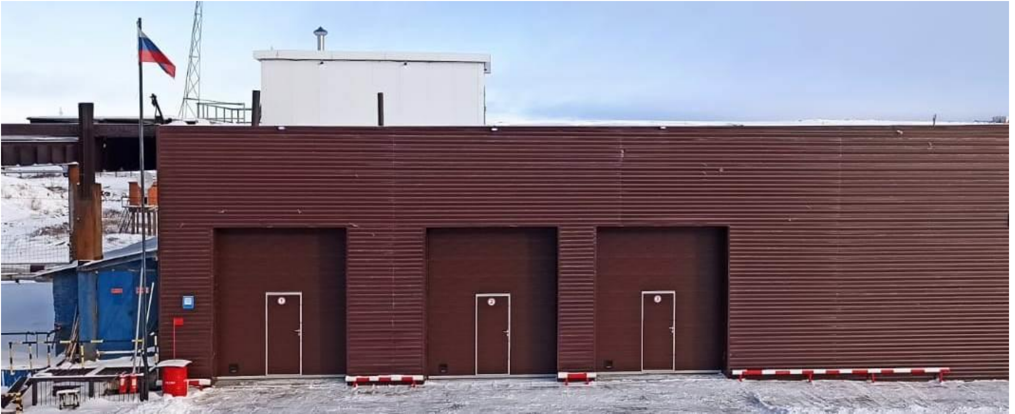
Photo of the building (front)
