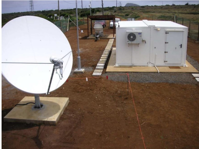
Figure 54: Lightning protection of a radionuclide monitoring station by a metallic tower providing protected volume for the satellite antenna and equipment container
