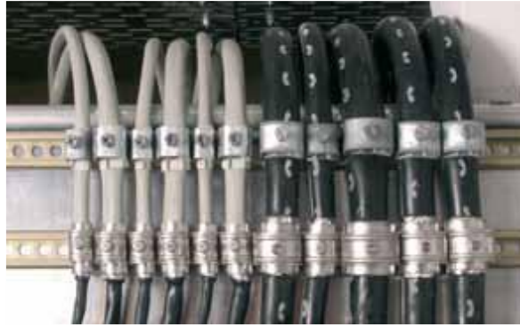
Figure 36: Shield connection system capable of carrying lightning currents
