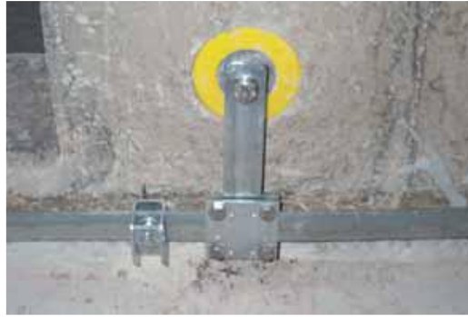
Figure 18: Connection of the ring equipotential bonding bar with the equipotential bonding network via fixed earthing point
